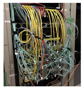
Figure 4.8: Photograph of ONSEN system installed at KEK. Optical cables in light blue are routed to patch panels that connect to EB2 and DHH. Ethernet cables in yellow and red connect to a switch above for slow control.
